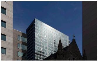
Gensler's redesign uplifts the exterior and lobby spaces, creates 13,000 square feet of street-level retail, and adds a 7,000 square-foot rooftop penthouse space. In a design-build process with an exterior façade contractor, the 24-story tower was fully reclad in glass and aluminum to refresh its appearance. Previous four-foot-high strip windows were replaced with floor-to-ceiling window glass,
