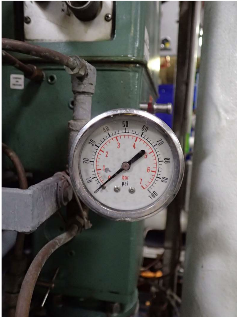
Photograph 48. - “B” Engine Governor Control Air Inlet Plumbing and Pressure Gauge
