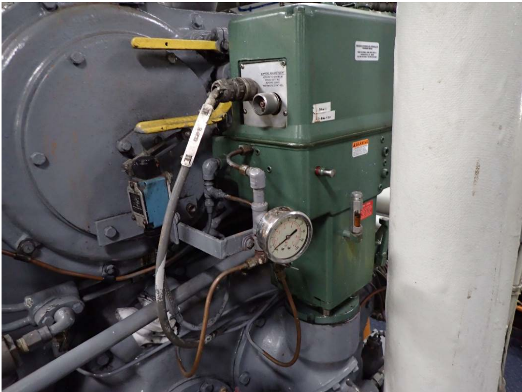
Photograph 56. - "A" Engine Governor Control Air Inlet Plumbing and Pressure Gauge
